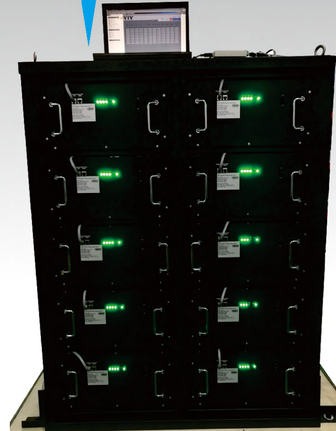
P.R Commercial Storage Demo: 52KWH Battery Storage System
